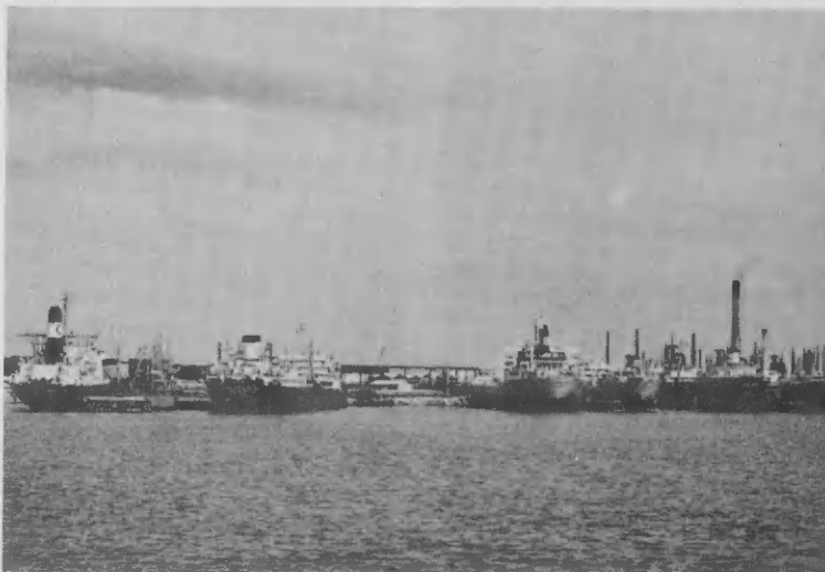
Harbor, looking east. Piers are equipped with modern, all metal loading arms. Piernan, cu brazanan di carga di metal.
